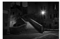
Bridge at Campo San Bolo
